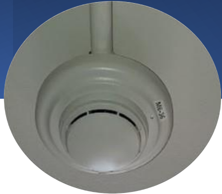
Typical Suite Smoke Detector
